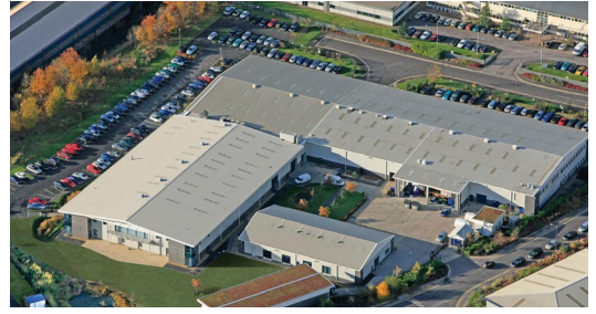
AESSEAL plc Group Headquarters, Rotherham, UK.
